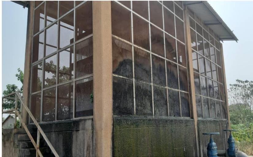
**Fig. 3. The Aeration chamber at the water treatment process at BWTP**
