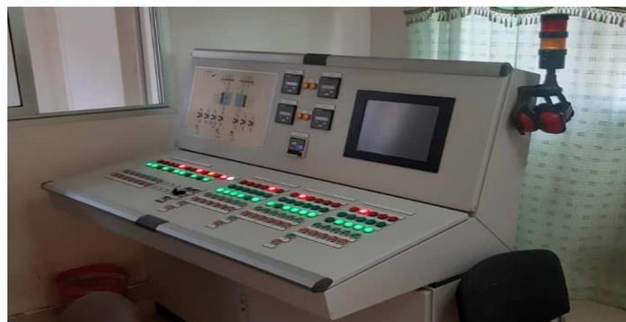
Fig. 2. Central Control Panel (CCP) installed at BWTP
